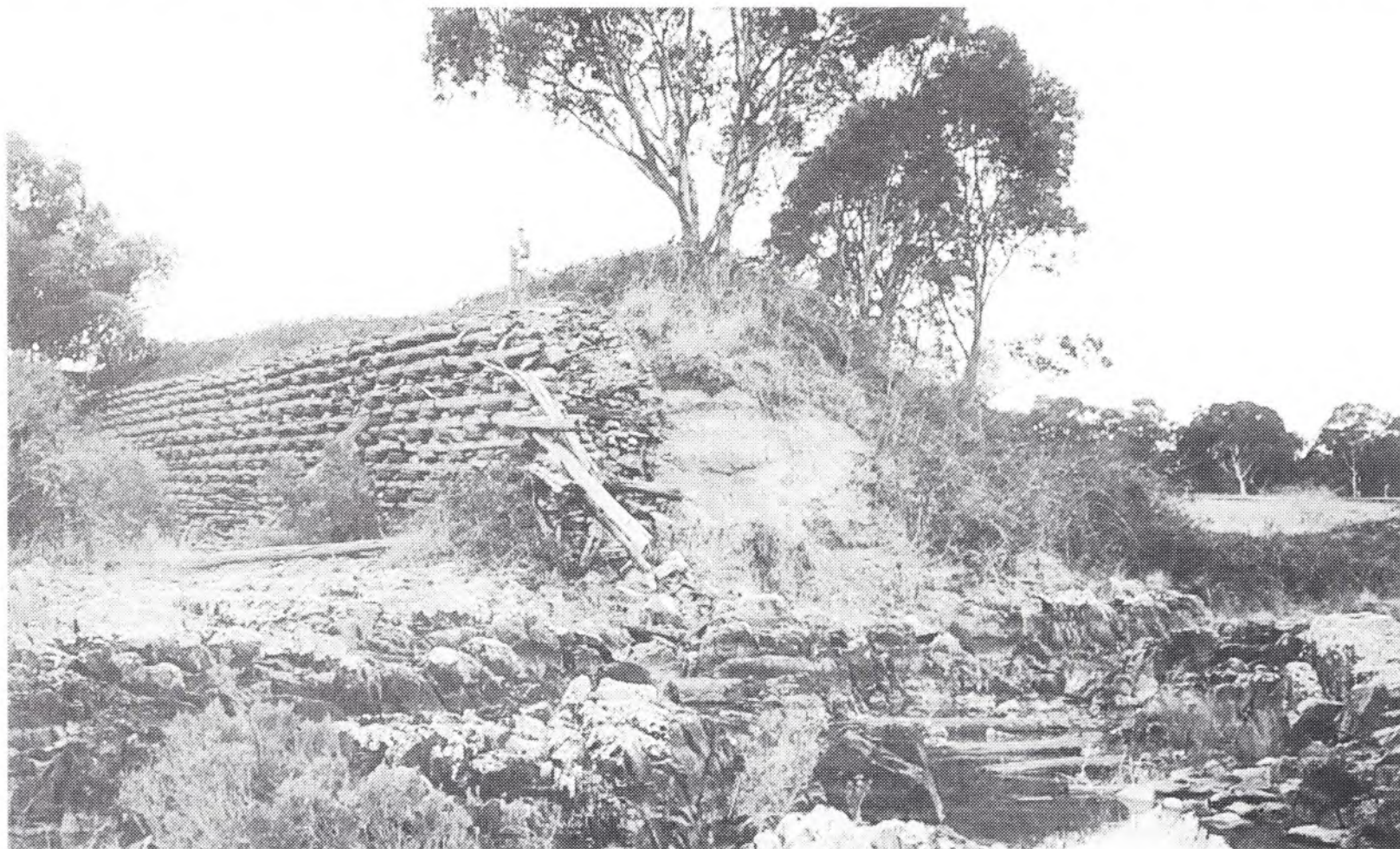
The remains of the larger Moredun dam are still impressive, despite being breached. Photographer K. Wiedemann.
